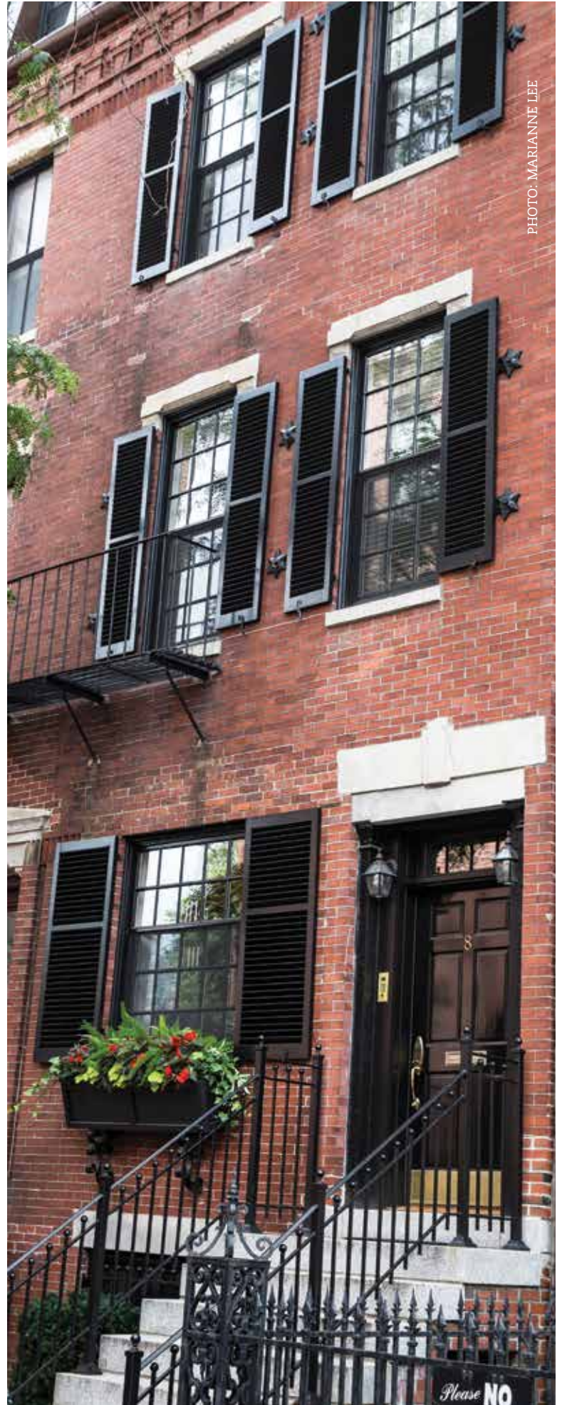
Seaport Shutter's Olde Style shutters grace a Beacon Hill brownstone.
